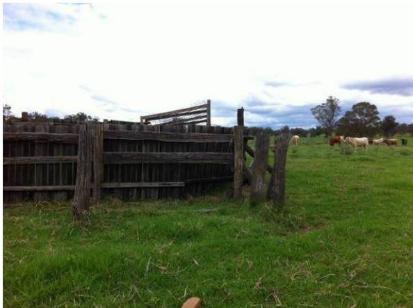
Figure 22: Existing timber posts located on corner, and reused for stock pens.
