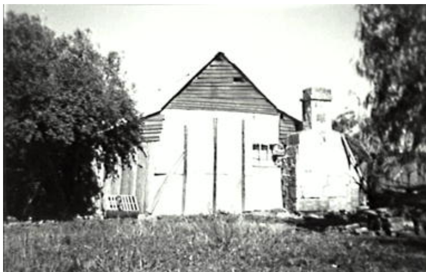
Figure A4: Side view of "Hillsborough" Chimneys c1980. Kingston Collection (Campbelltown City Library. Local Studies Collection).
