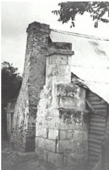
Figure A2: Side view of "Hillsborough" Chimneys. Campbelltown & Airs Historical Society.
